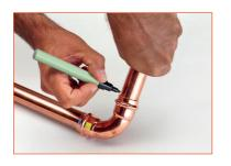
4) **Insert the pipe into the fitting** as far as the bottom, while turning it slightly. Mark the pipe with a pen in order to check any sliding before or during the pressing.
