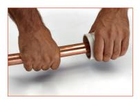
2) **Carefully deburr the pipe**, both internally and externally, as a possible residual burr could damage the O-rings and compromise the tightness of the connection.
