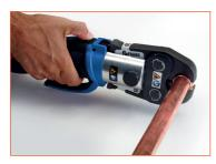
6) **Set the pressing tool** properly and make sure that the toroidal chamber is inside the jaws. Carry out the pressing until the jaws touch each other.
